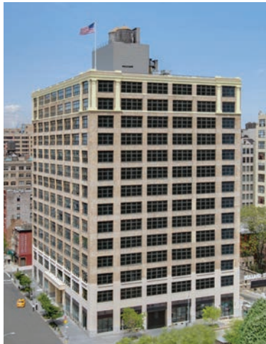
Top: 255 Greenwich Street Bottom: 250 Hudson Street
