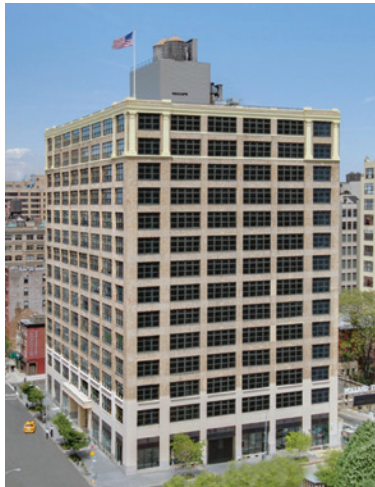
Top: 255 Greenwich Street Bottom: 250 Hudson Street
